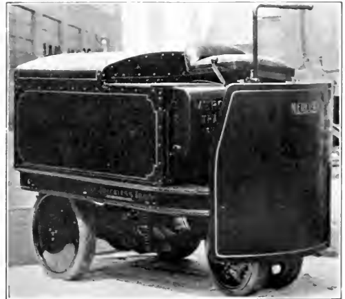
FIG. 1 MERCURY TYPE H INTERNAL GEAR DRIVE TRACTOR
